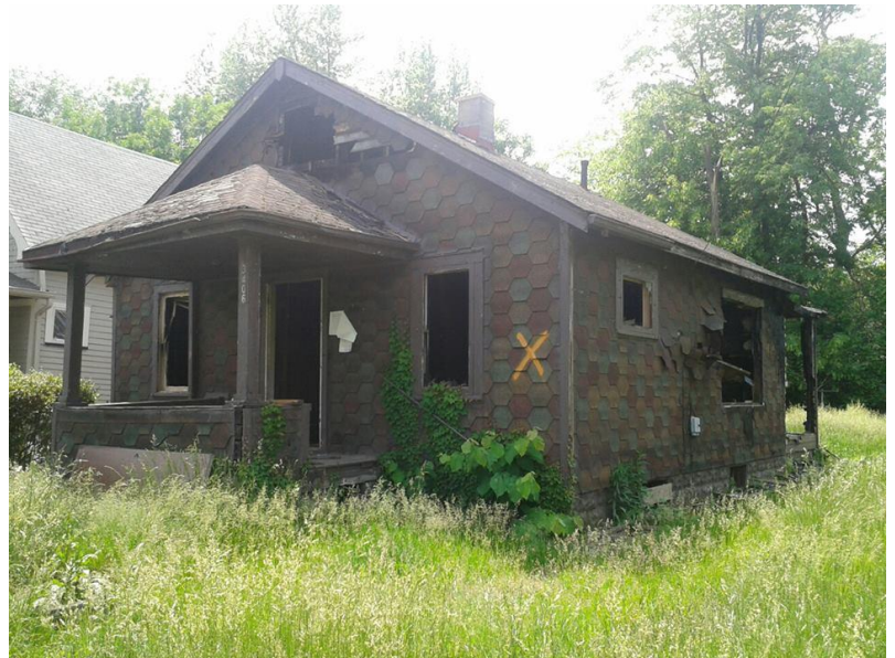
Photo: Vacant house in Cleveland's Slavic Village
